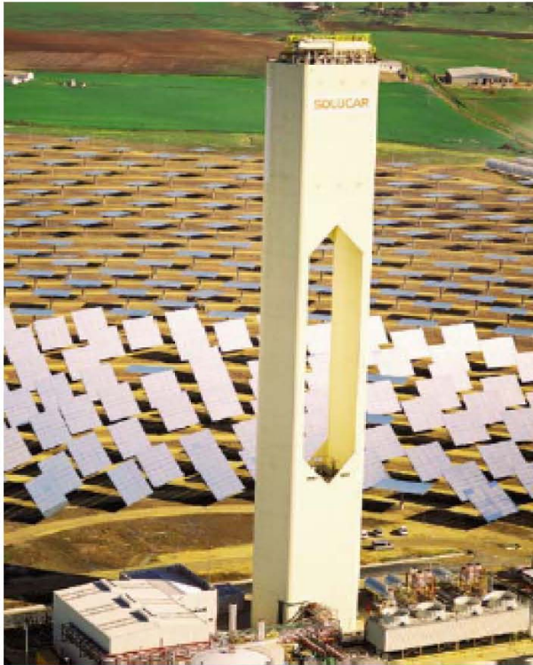
Figure 1: Above, power tower pilot project, pioneered in the U.S. (Barstow, CA) and (left) commercial unit under development by Abengoa called PS10, an 11 MW plant in Sevilla Spain (photo credit: Abengoa Solar). Bottom left, Stirling Dish/Engine, Center SEGS trough plants, Right, Compact Linear Fresnel Reflector.
