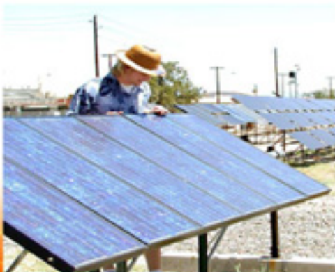
Flat panel photovoltaic (PV)
